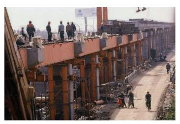
Fig. 6. Construction of Transrapid infrastructure in Shanghai [12]
